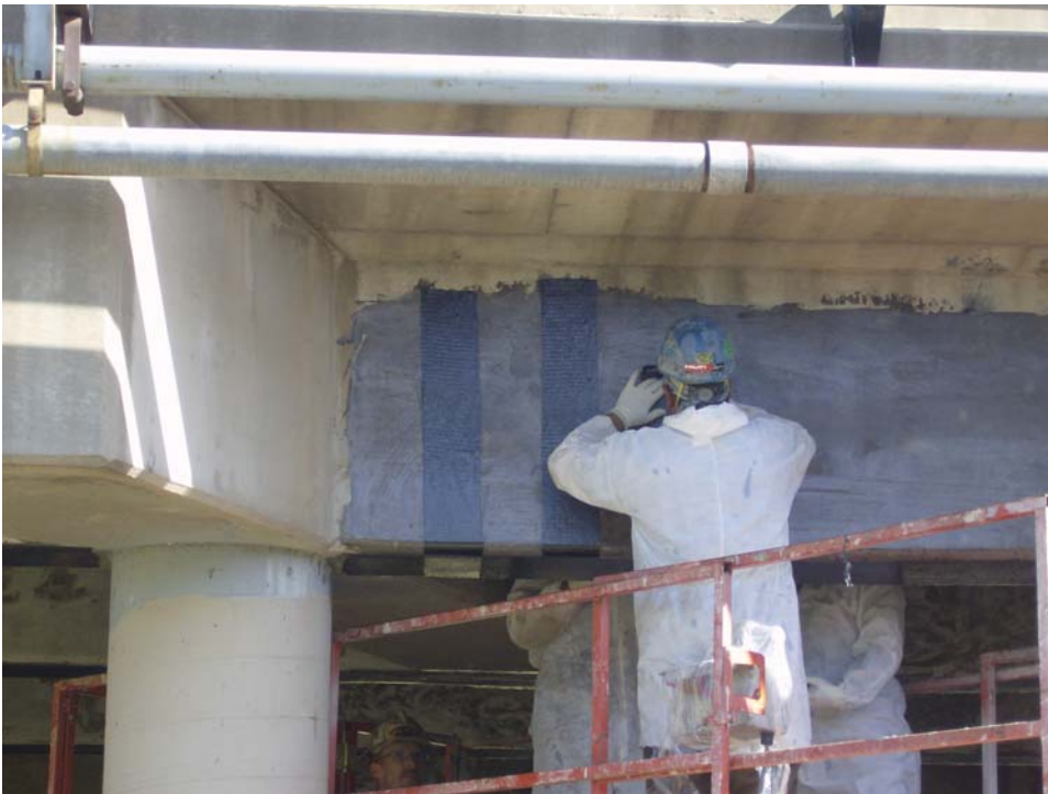
CFRP U-wraps installed on T-beams of the Thunderbird Road Bridge.
