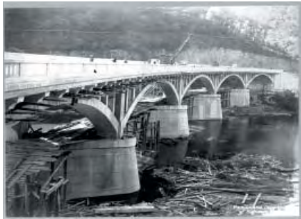
Figure 3 – Original Construction – 1935 (Photo courtesy of HAER)
