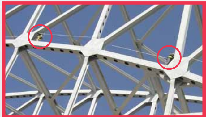
Gannett Fleming's inspection team free climbing the main through-truss spans
