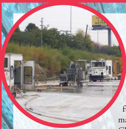
Drilling and grouting operations at the McCook Reservoir.
